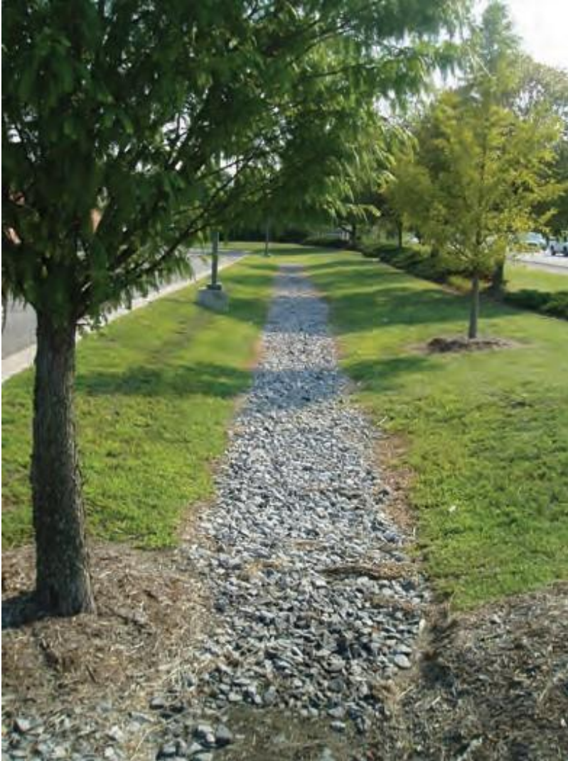
Figure 4.16. Infiltration practice in median strip.
