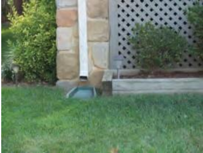
Figure 4.32. Rooftop disconnection (photo: Center for Watershed Protection, Inc.)
